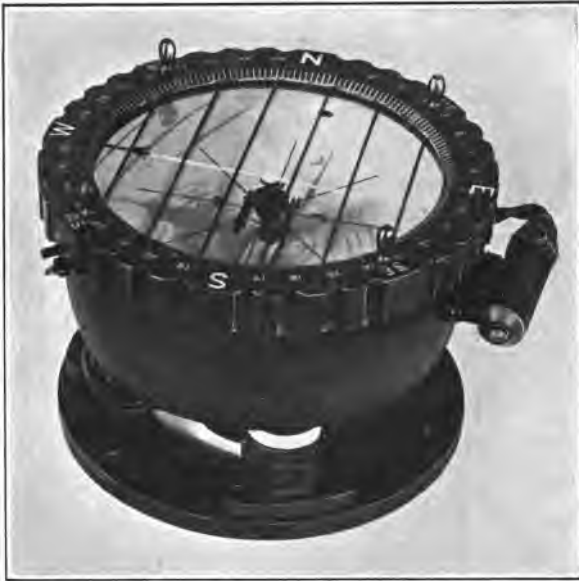
FIG. 18.—A.C.O. aperiodic compass—6/18 (Bennett).
