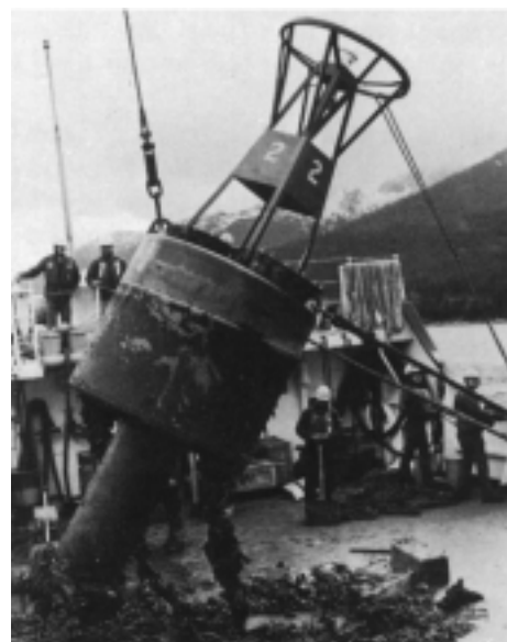
Figure 509. Buoy showing counterweight.
