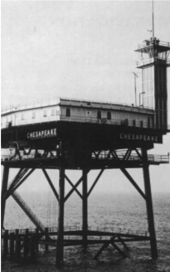
Figure 501a. Typical offshore light station.
