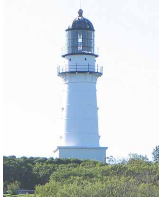
Figure 712. Typical Major Light.
