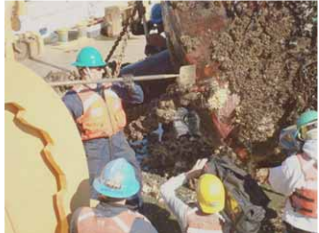
Figure 709. USCG removing marine growth from a buoy.
